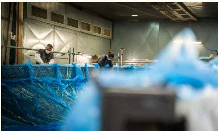
Chantier Multiplast à Vannes, France (c). Yann Riou
